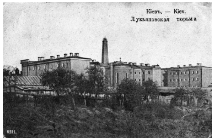
Lukyanovka Prison as shown on a postcard around 1900. It looks pretty much the same today, except that the city has grown up all around it. (Photo credit: Wikipedia)
